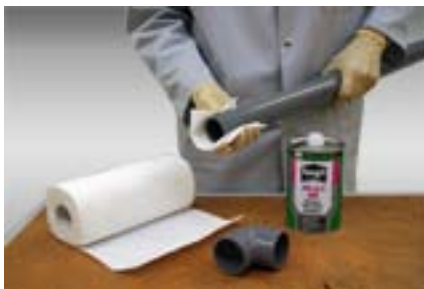
Cleaning the pipe and socket
